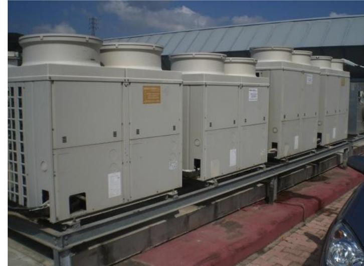
$17 \times 2 \text{ kW} + 21,5 \times 2 \text{ kW} = 77 \text{ kW}$  frigoriferi
